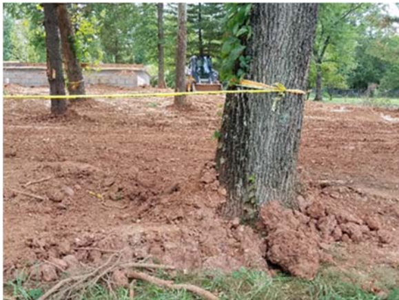
Figure 3: Root and soil disturbance
