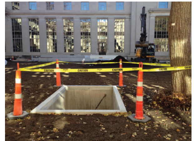
To install this area-way at M.I.T. required diligent tree protection, and intensive excavation using an AirSpade and root pruning by a trained arborist. (Image courtesy of SSA.)
