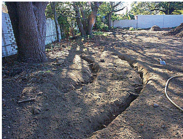
Trenches are being located around this existing tree to accommodate an electrical conduit.
