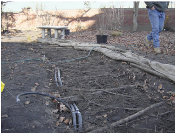
At the Radcliffe Institute, the foundation for a new path was excavated using an AirSpade. Irrigation lines were snaked through the exposed roots, and minimal root pruning was completed before installing a gravel root barrier and the top course of stone dust pavement. (Image courtesy of SSA.)
