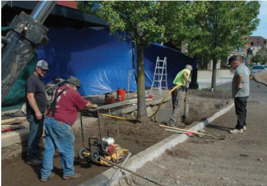
Installation of a new paving system for ginkgo street trees. At the right of the photo, an arborist excavates highly compacted sandy loam soil that had supported brick pavement for over 20 years. At left, the contractor finishes installation of an engineered sand based structural soil, which is to bear the load of new pavement.
