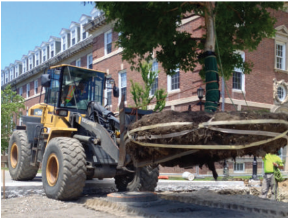
This tree at Williams College was bare rooted using an AirSpade and transplanted as part of a new quad construction project. (Image courtesy of SSA.)
